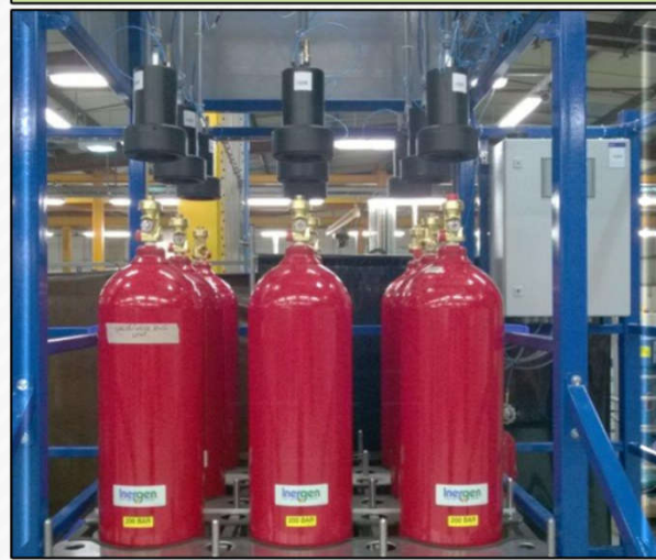
Leak Test (IG)
